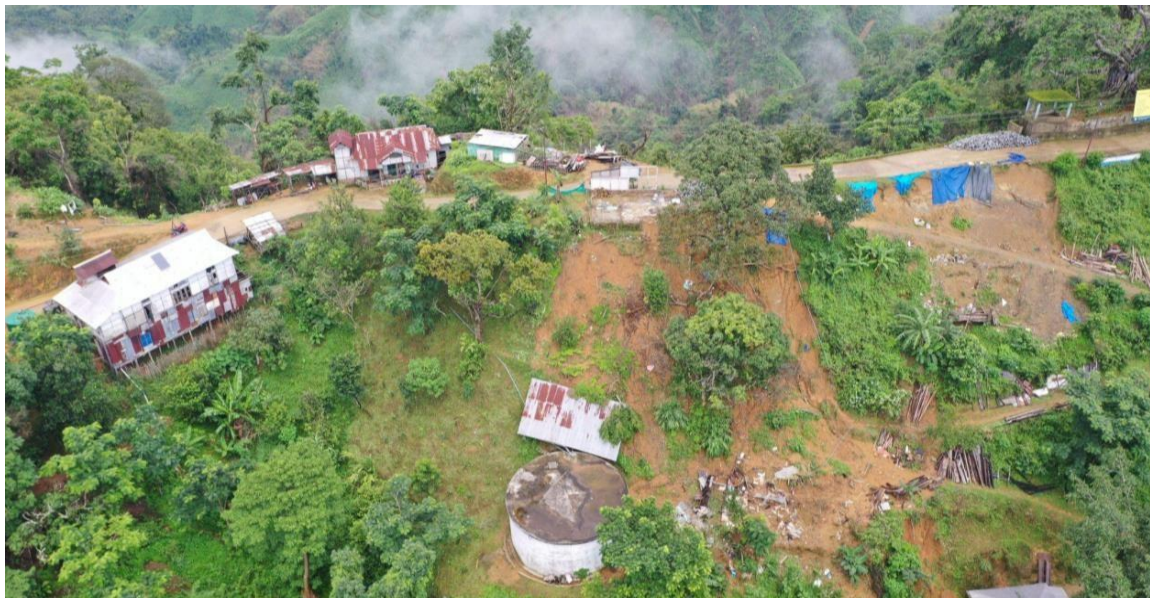
Figure 5 Aerial view of village affected by landslide
