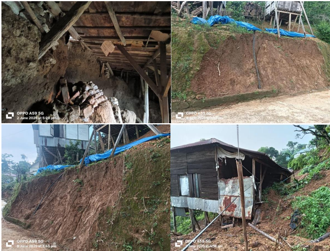
Figure 4 Houses affected by landslides
